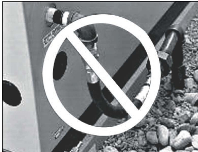
Figure 5-4. Incorrect Routing of Flexible Hose
