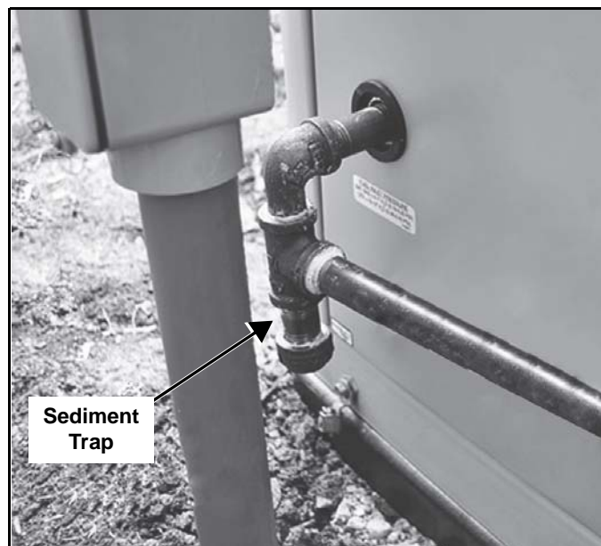
Figure 5-3. Sediment Trap
